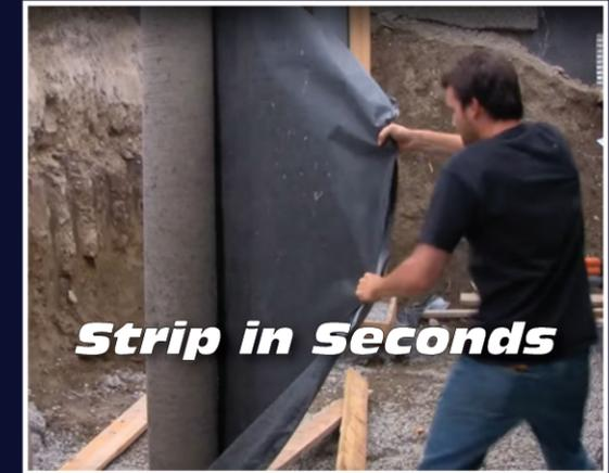
Pull on the alignment tab, Fast-Tube™ strips in seconds. Polyethylene does not bond to concrete.
